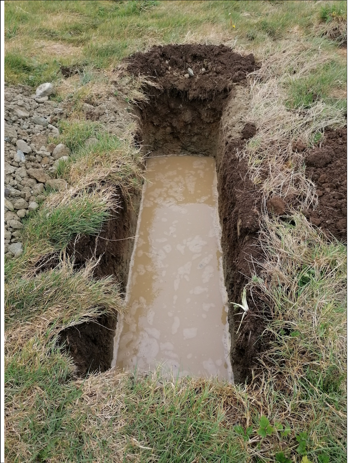
Plate 11: SA TP106 terminated at 1.30m
