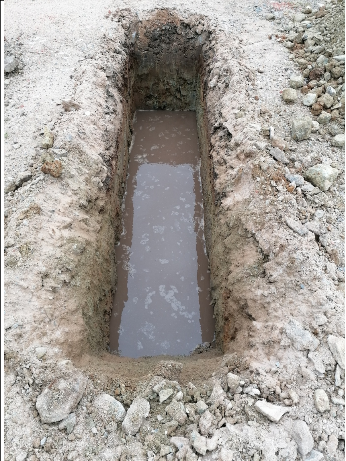
Plate 7: SA TP104 terminated at 1.20m
