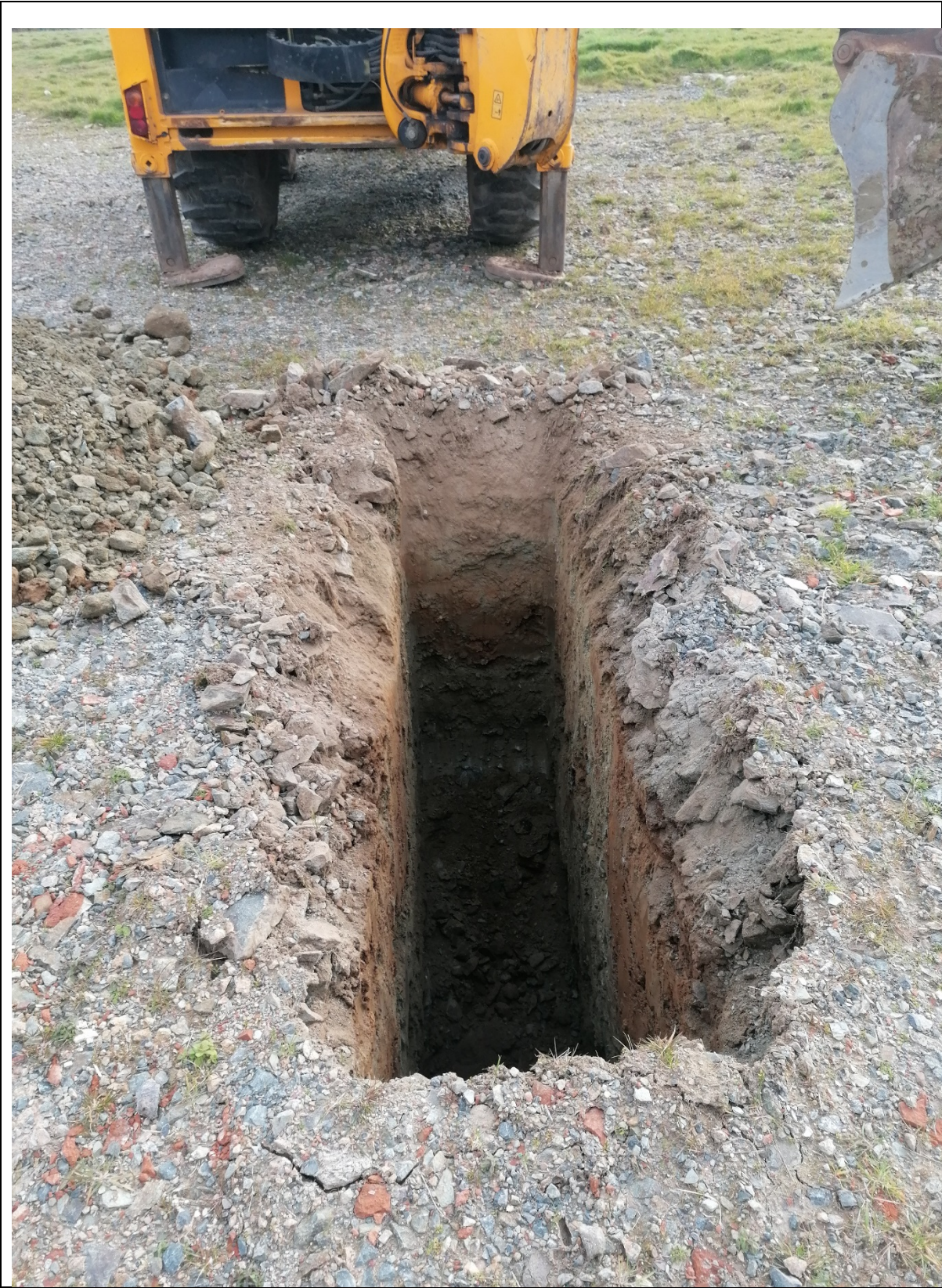
Plate 1: TP101 terminated at a depth of 2.50m
